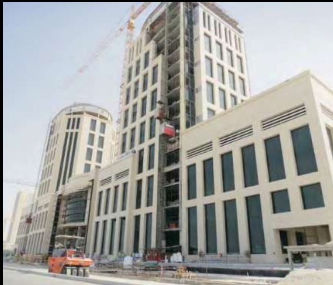
External Building Cladding - Bahrain
